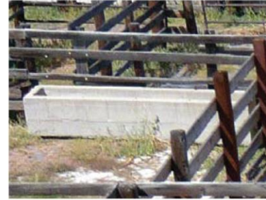
NWC: Historic concrete water trough in the Yards
