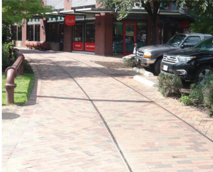
Pearl Brewery District: Historic rails define new pedestrian walkway
