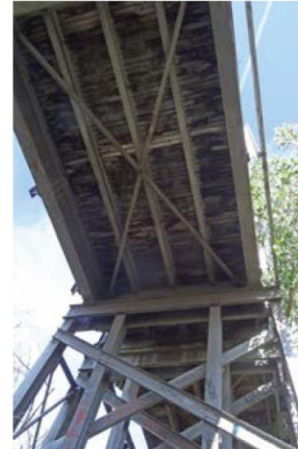
NWC: Historic sheep bridge over the Platte River
