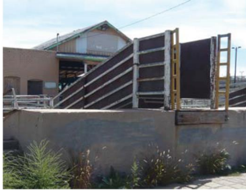
NWC: Concrete and metal loading ramp
