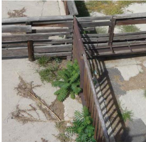
NWC: Wood and metal pen structures; concrete paving
