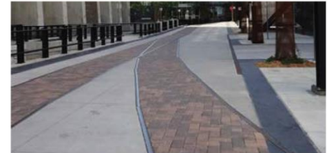
Minneapolis: Rails are highlighted with brick pavers to reflect historic circulation patterns
