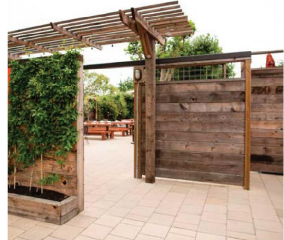
HopMonk Beer Garden: Reclaimed wood planks used to frame and shelter an outdoor seating area
